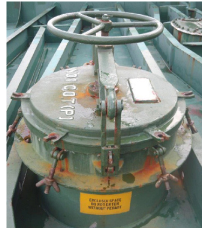
Figure 4: COT No. 1P access hatch showing warning label "Enclosed Space Do Not Enter Without Permit."
