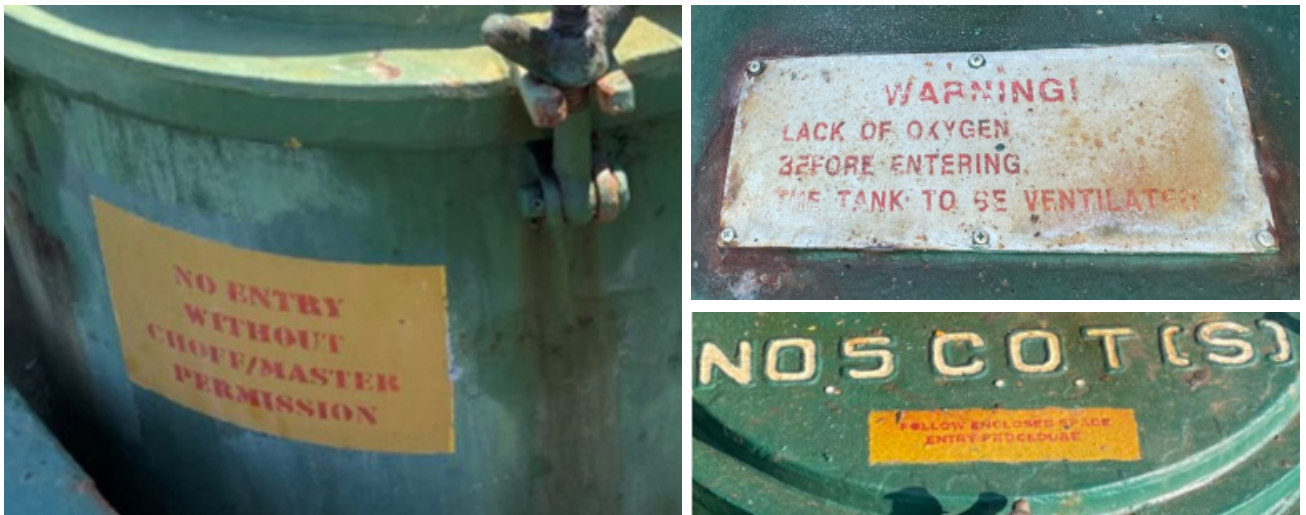
Figure 2: COT No. 5S tank access hatch cover warning signage.
