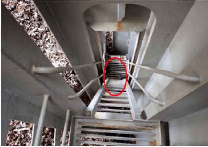
Figure 1: Cargo Hold No.1 aft access ladder. The red circle indicates where the C/E, ETO, and Fitter were located at the bottom of the inclined ladder on the intermediate platform. The cargo of scrap metal is visible in the hold.
